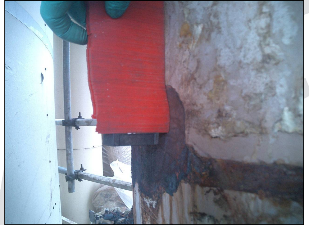
External corrosion on a vertical pipeline. Located at a circumferential insulation clamp.
